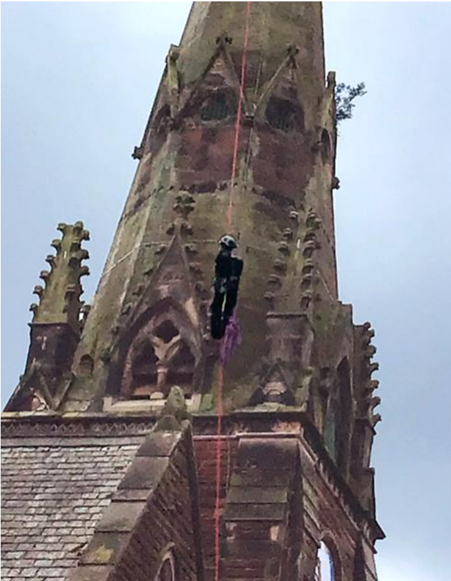
1. Before work started—see the vegetation!
